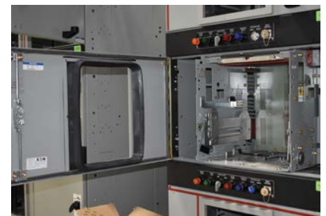
Bellows and Two-Point Door Latch
