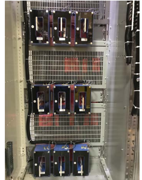
Optional Bus Compartment and Vertical Section Barriers (feeder CTs shown)
